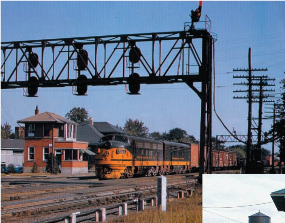
Left: RU cabin at Russel had a non-standard addition on the front for yard clerks.
