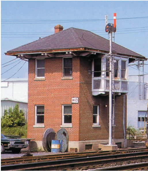
HO Cabin at the west end of Huntington - a classic example of a C&O Standard Cabin brick cabin.
